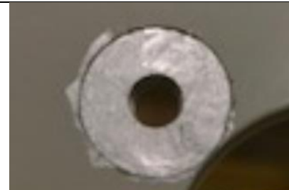
Figure 5 – Surfaces that may exhibit some over paint from masking removal are acceptable if they do not exceed 1/4”.
