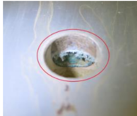
Figure 42 – Discolored Plating (Green)
